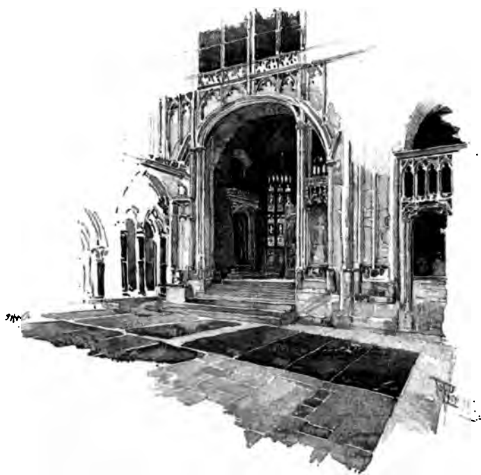
ST. PAUL'S CHAPEL, NORTH ARM OF TRANSEPT.
